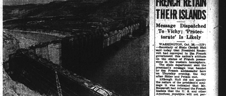
Most of the 16,000,000 cubic yards of concrete that will form Grand Coulee dam on the Columbia river are in place now, as the huge dam nears completion. In the foreground of this view is the wing dam, which will form the front wall and a base of the pumping plant to built later.
